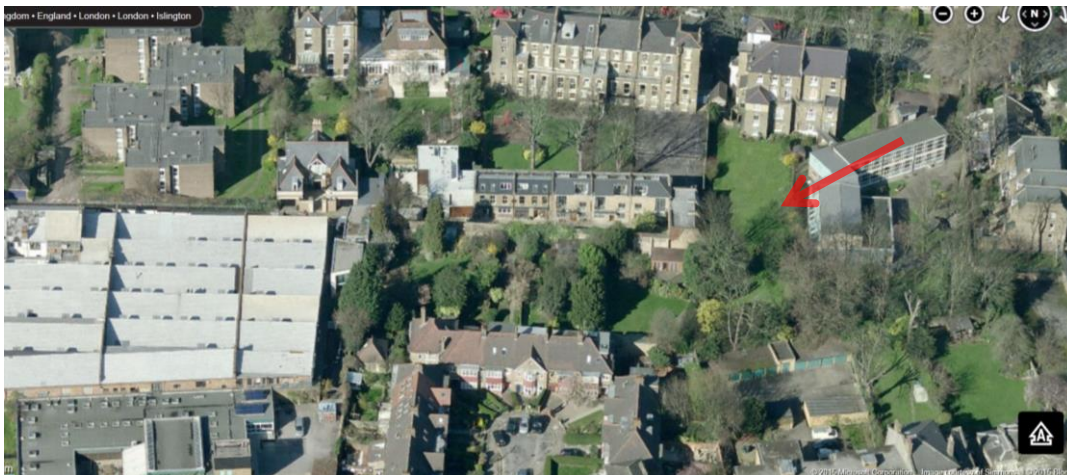
Image 1: Aerial view of the application site
