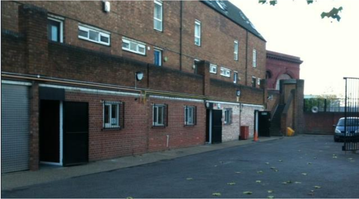
Image 1: View of office space (previous undercroft)
