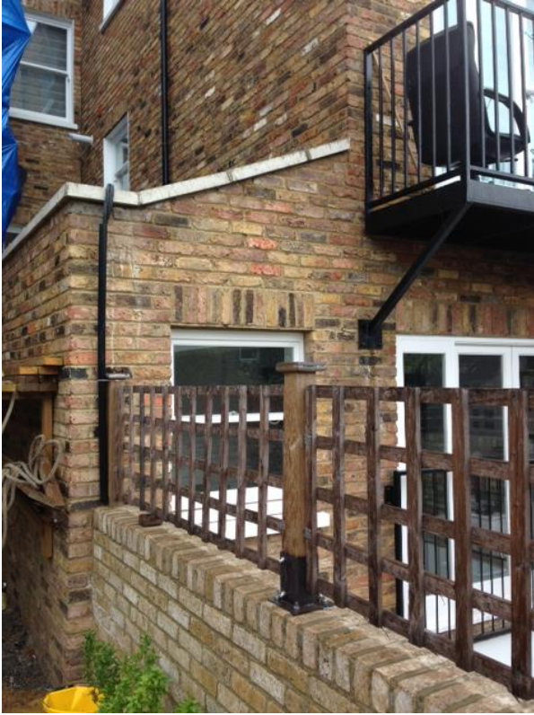
Image 3: View looking to the rear of 70 Hanley Road
